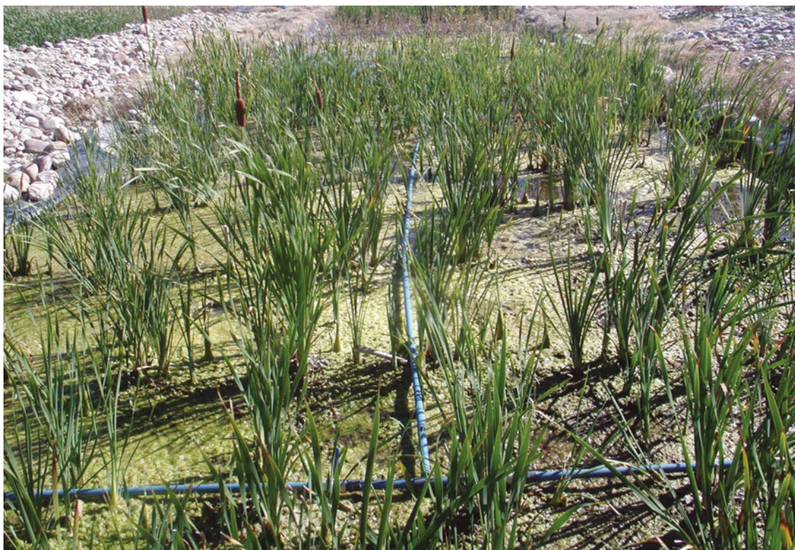
FIGURE 1: Constructed wetland at Goudini with liquid capacity of 56.7 cubic metres used to treat 4.05 cubic metres of wastewater per day at a retention time of 14 days.
